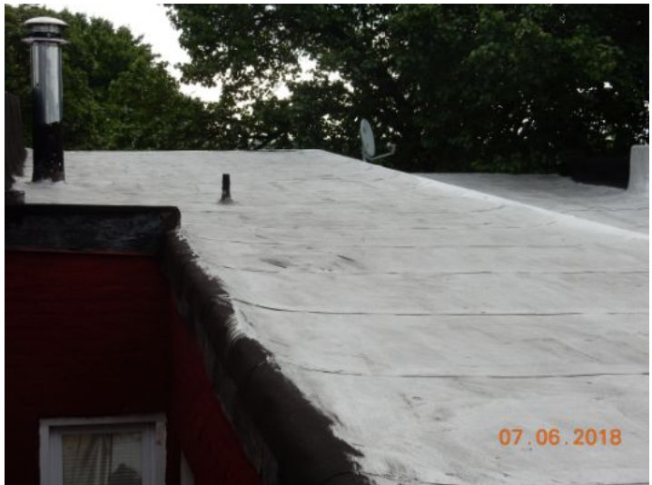
Modified bitumen (rubber) roofing
