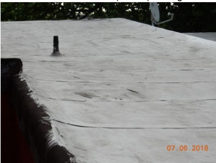
Modified bitumen (rubber) roofing
