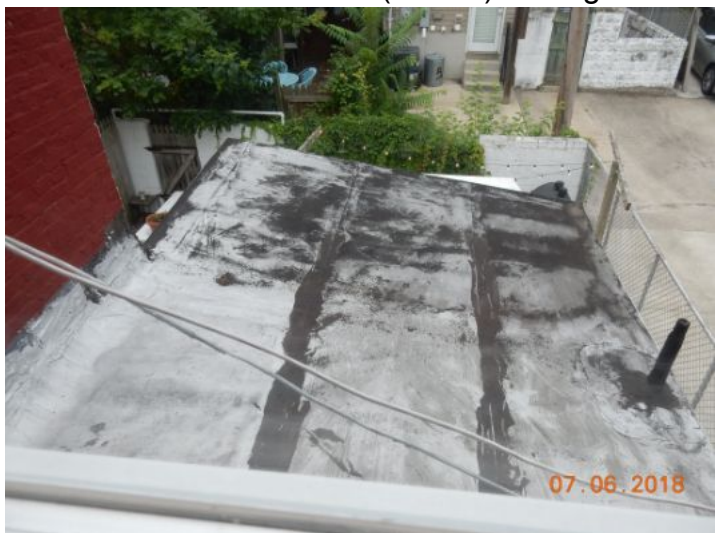
Modified bitumen (rubber) roofing
