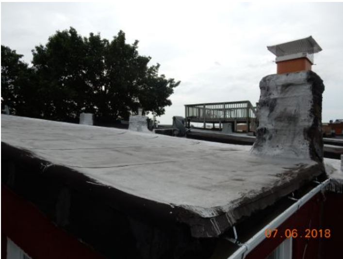
Modified bitumen (rubber) roofing
