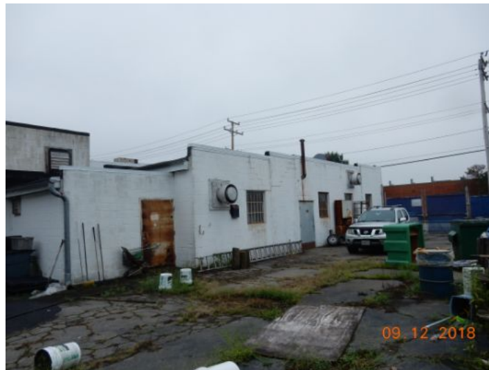
Parking, loading area
