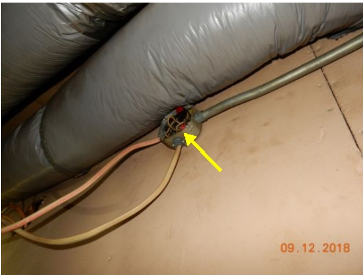
Open junction box 2nd floor
