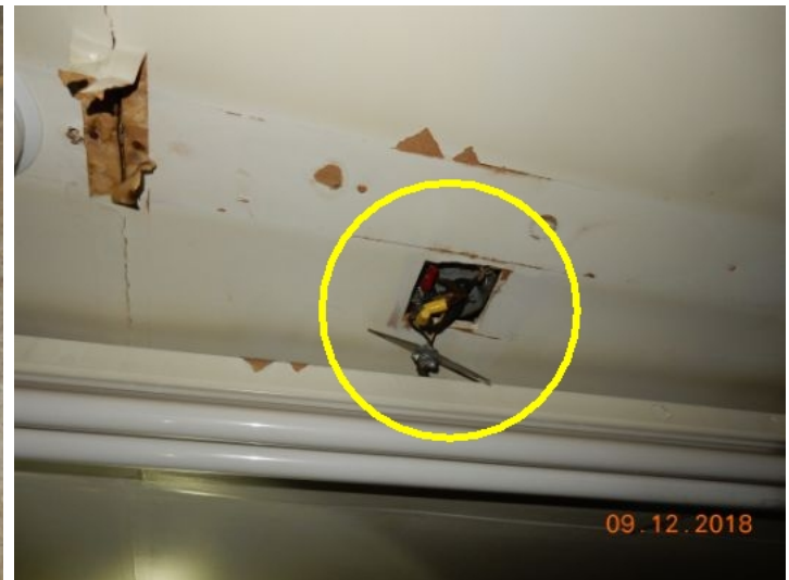
Open junction box - 2nd floor
