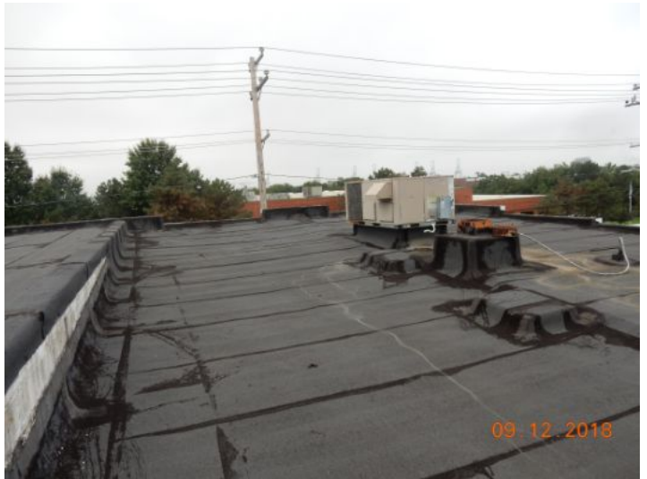
Typical roof view
