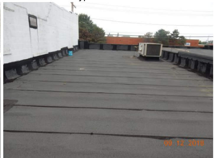
Typical roof view
