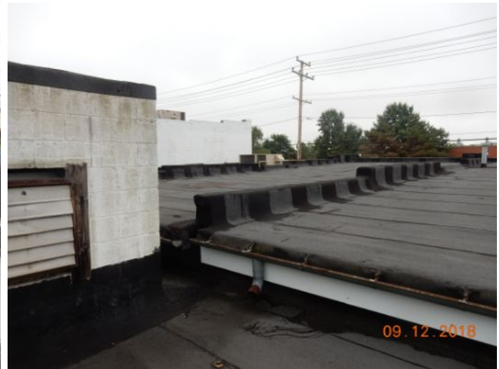
Typical roof view
