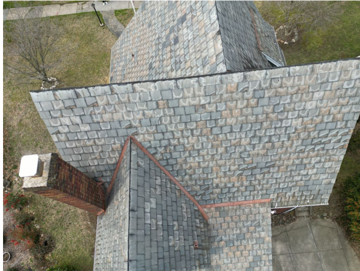
Slate roofing in good condition.
