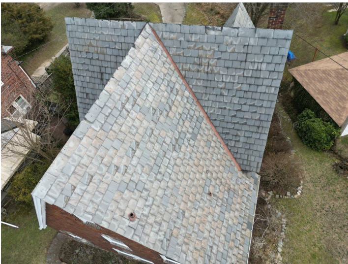
Slate roofing in good condition.
