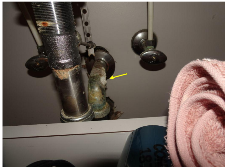
Replace corroded sink traps as preventive maintenance
