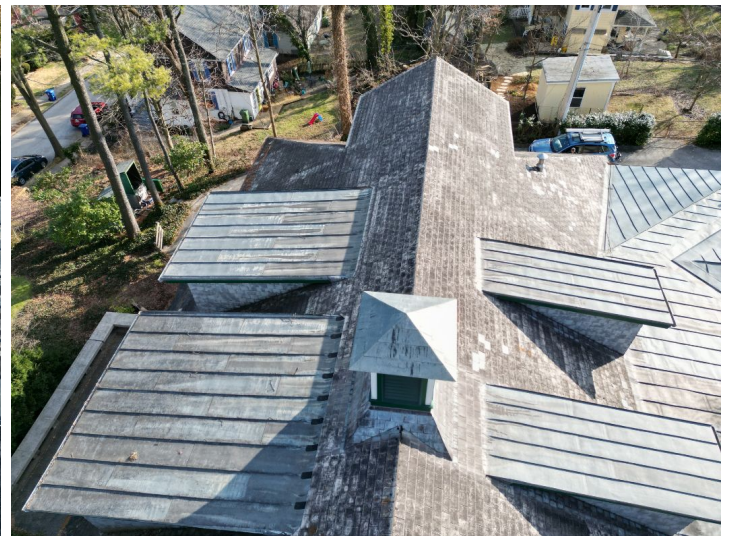
Metal and shingle roofing
