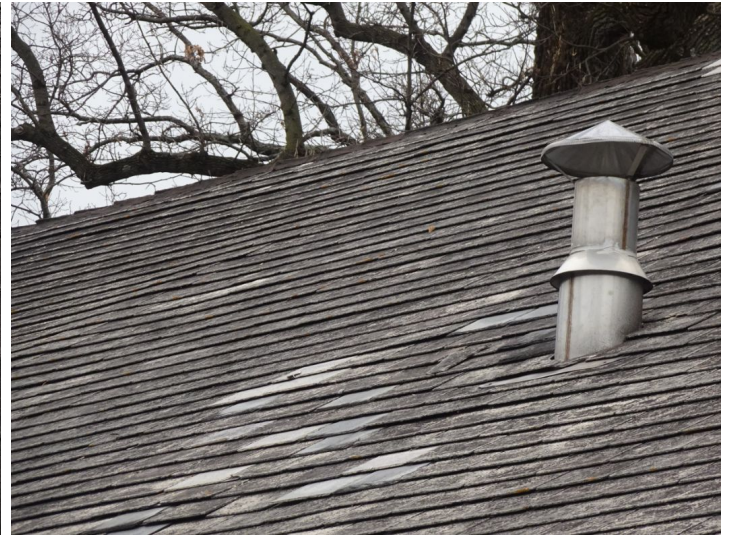
Shingle roofing in serviceable condition
