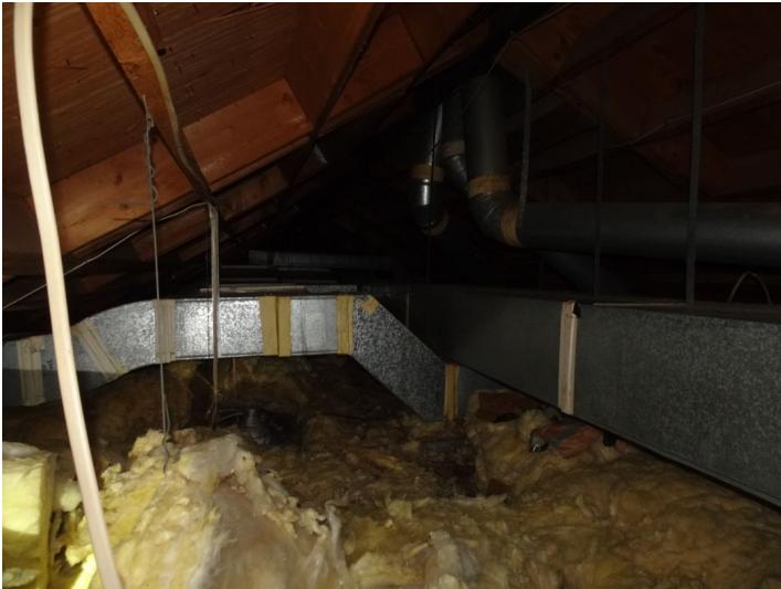
Attic insulation and framing.
