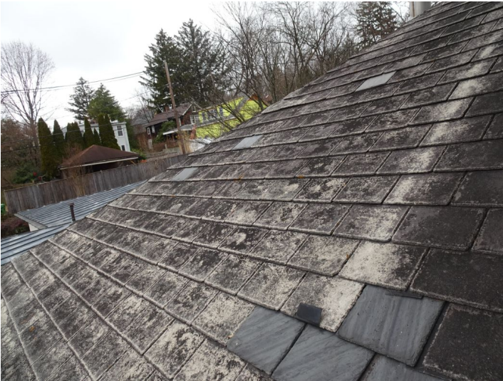
Shingle roofing in serviceable condition
