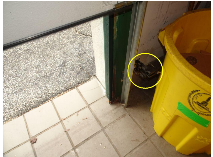
Garage vehicle door photo electric sensors are mounted higher than normal. Install 6" above floor.
