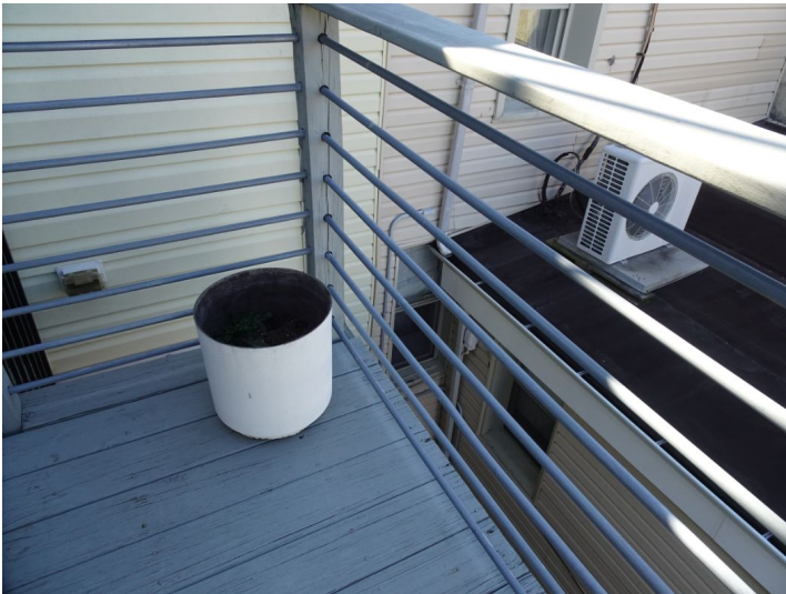
Hand railings are climable. This is not considered child safe. Modify to promote safety
