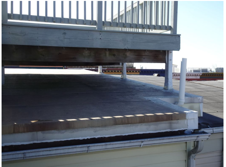
Deck structure is sound.
