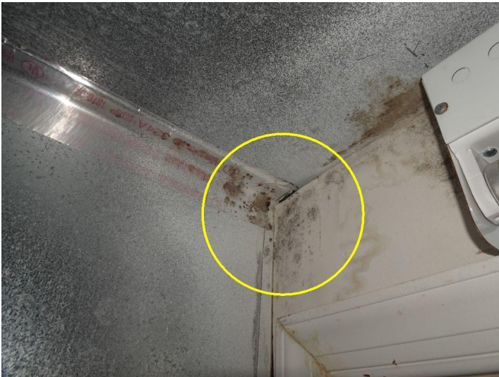
Possible organic substance noted. Utility room - 2nd floor. You may wish to test for mold.
