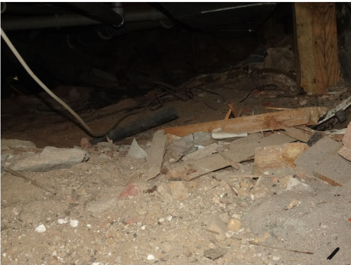
Remove debris in crawlspace.
