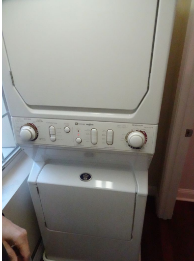
Washing machine and dryer operational
